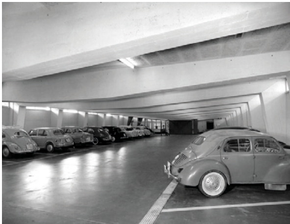
Le garage © Archives de la Vaudoise Assurances
